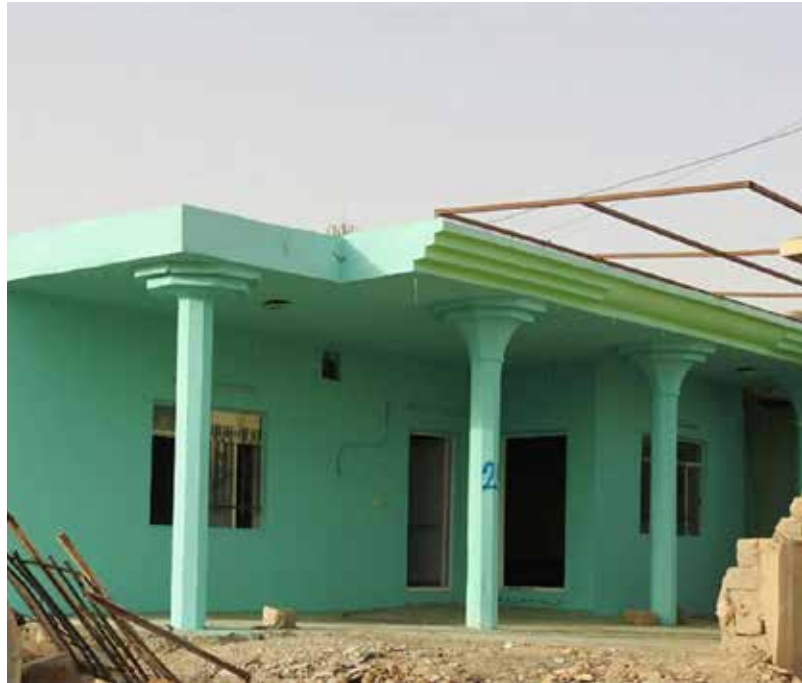
Top Left Image: Before (damaged house). Top Right Image: After (Rehabilitated house).
